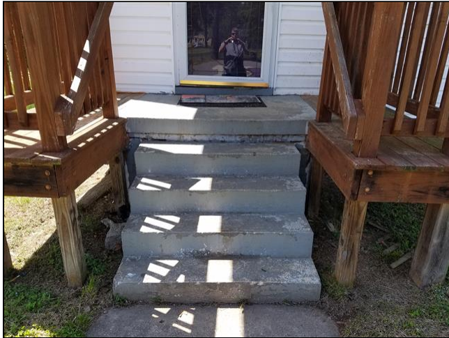
2.4 Item 1(Picture) Partial handrails at front
