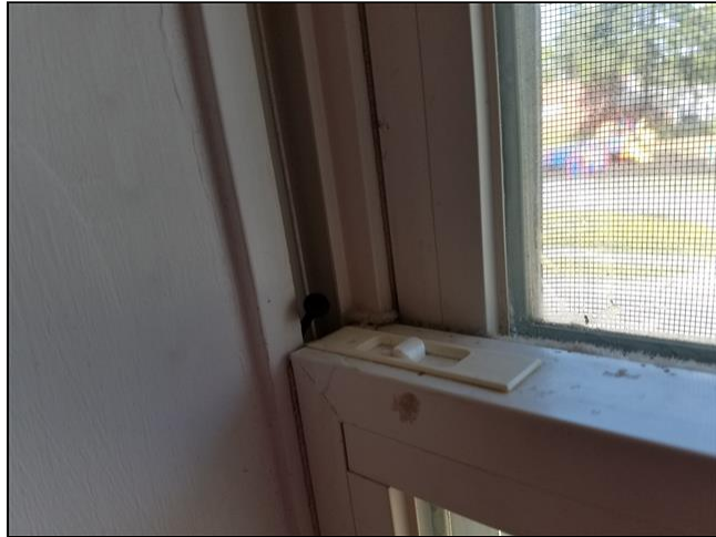
3.6 Item 1(Picture) Front bedroom window nailed shut 3.6 Item 2(Picture) Broken window in kitchen (1) Front bedroom window is nailed shut; doesn't properly operate.
