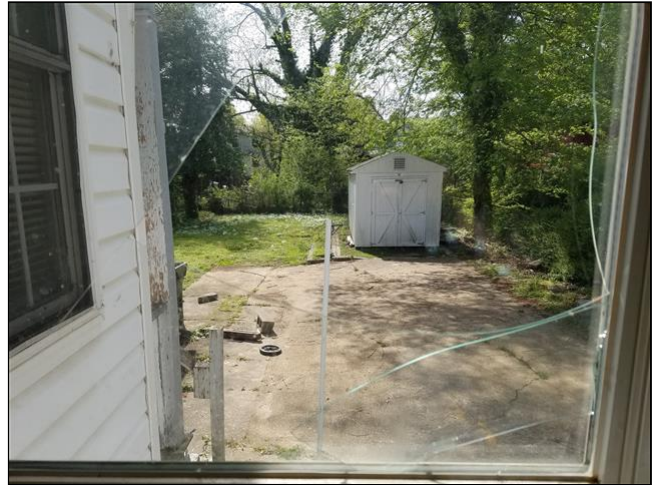
3.6 Item 1(Picture) Front bedroom window nailed shut 3.6 Item 2(Picture) Broken window in kitchen (1) Front bedroom window is nailed shut; doesn't properly operate.
